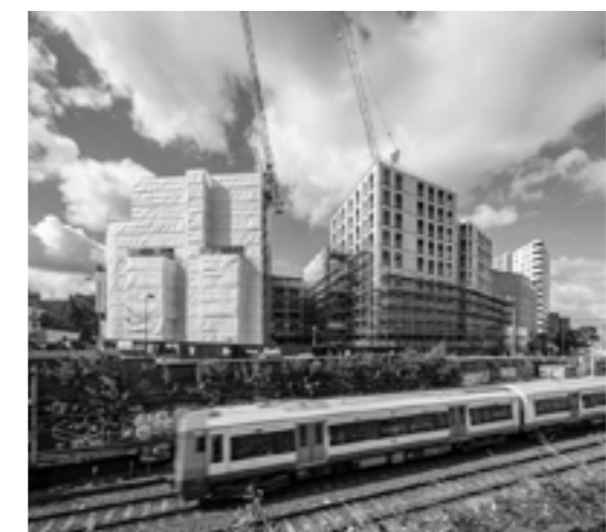
Project: Dalston Works Source: https://waughthistleton.com/dalston-works/
